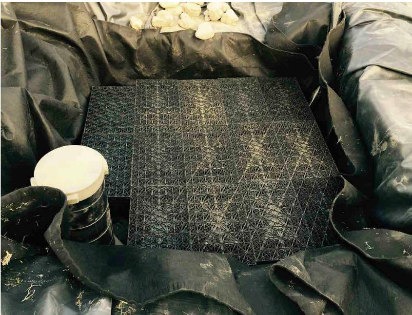
Completed basin with water storage block installed.
