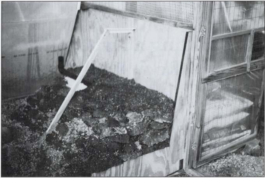
Construction of the hypertufa rock wall, showing treated plywood backing, irrigation pipe about to be buried, and painted hypertufa rocks. (Ev Whittemore)
