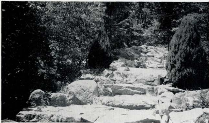
Rock stairway to prevent heavy rainfall from eroding driveway.
