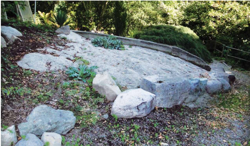
Site of tufa bed before construction
